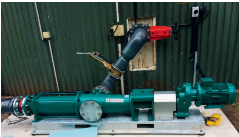
沼气项目中使用的螺杆泵 Eccentric screw pump in use in a biogas plant
