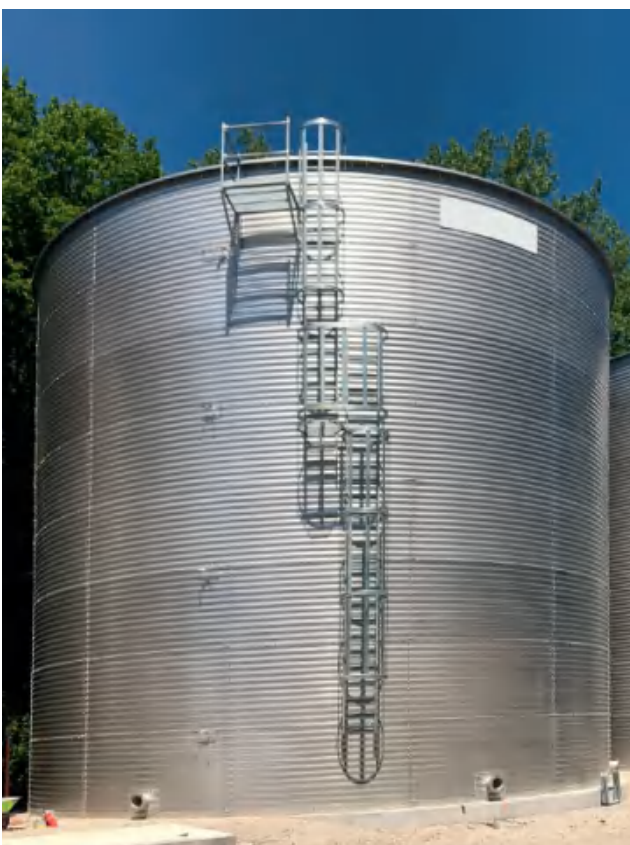
1.304 m 3 膨润土悬浊液储存罐（瑞士） 1,304 m 3 Bentonite suspension tank in Switzerland
