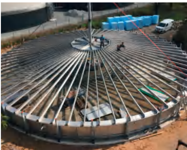
不锈钢屋顶的储存罐 Tanks with stainless steel roof construction
