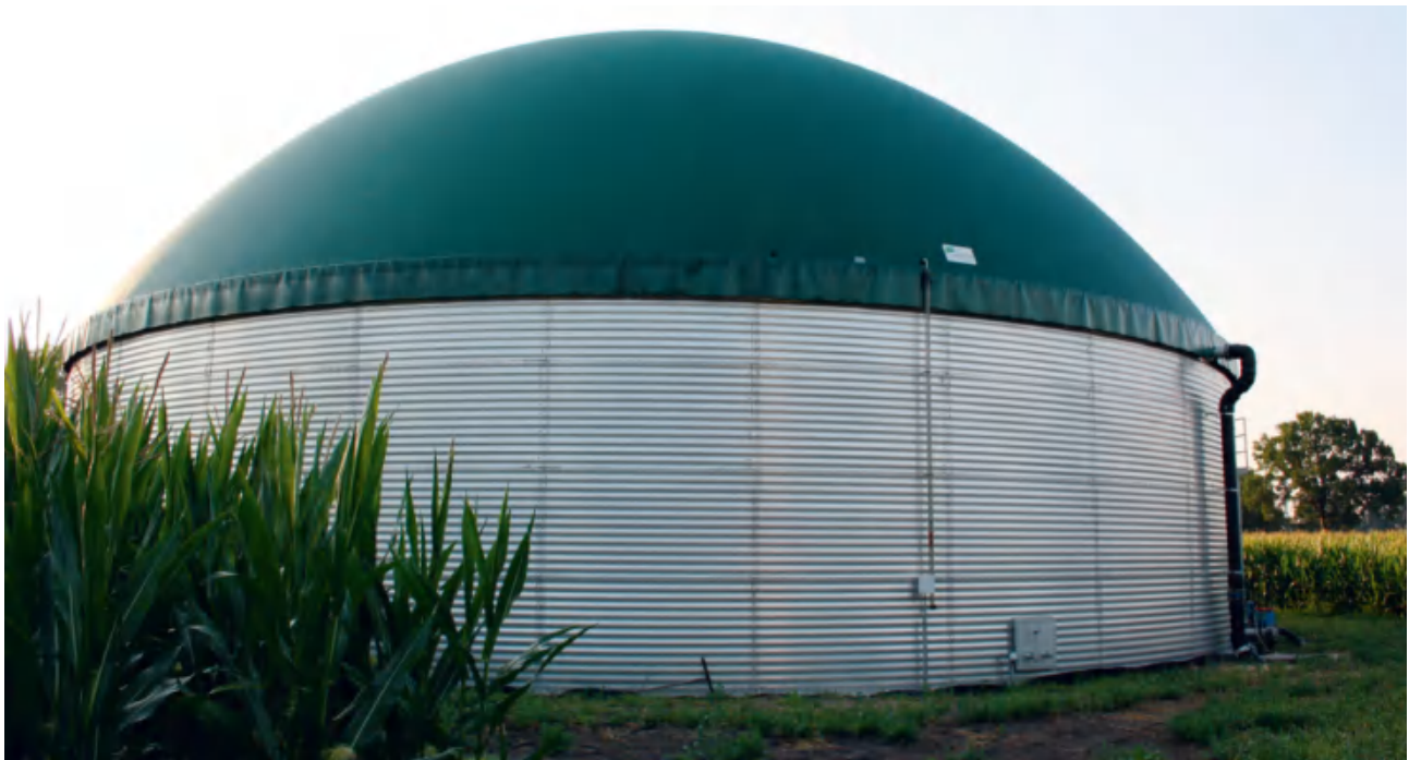
采用气密双膜屋顶的沼气发酵罐 | V4A biogas tanks with gas-tight double membrane roof
