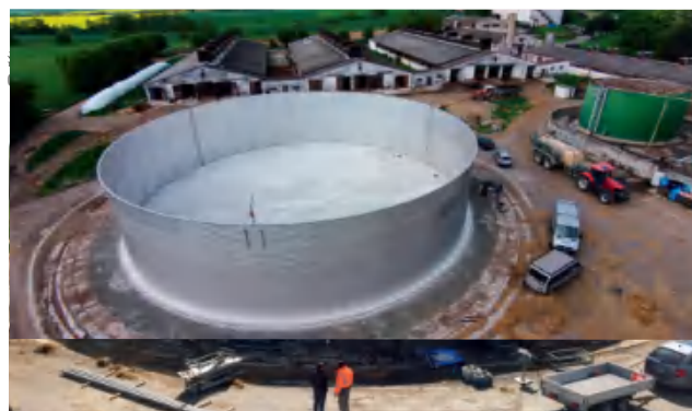
6,283 m 3 波纹不锈钢罐 (捷克共和国) 6,283 m 3 Corrugated steel tank in the Czech Republic
