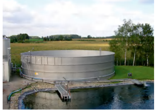
不锈钢污水罐 Stainless steel tank for waste water
