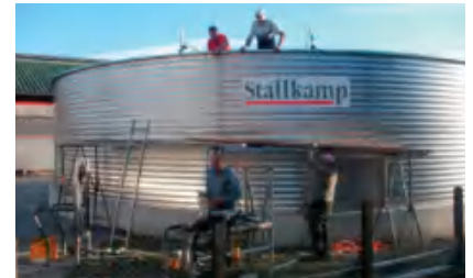
加高后的混凝土罐 Heightened concrete tanks
