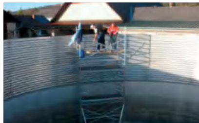
混凝土罐上加高的两圈罐 2. Ring on concrete tank
