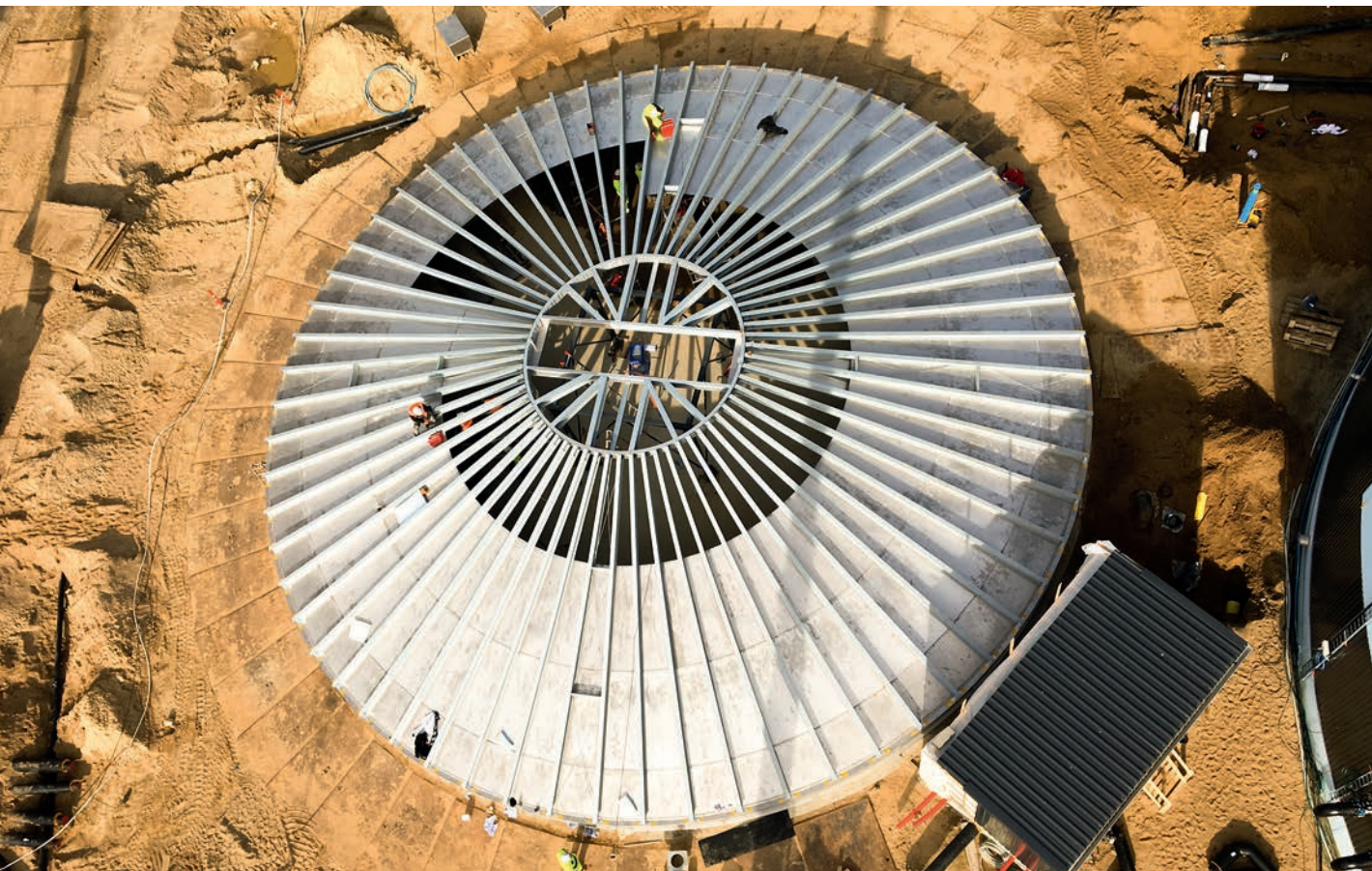
Montage des Edelstahldaches Assembly of stainless steel roof
