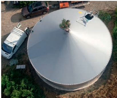
Membrandach von oben | Membrane roof from above
