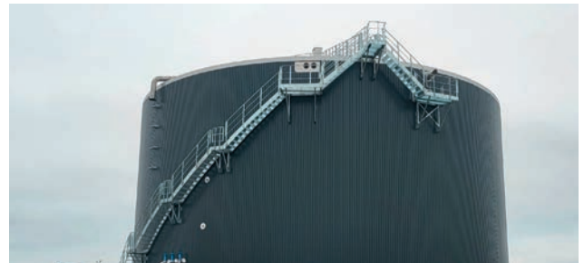
Tankmanteltreppe Tank Staircase
