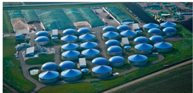
Fermenter, Nachgärer und Gärrestlager einer Biogasanlage Digester, secondary digester and end storage of digestate of a biogas plant
