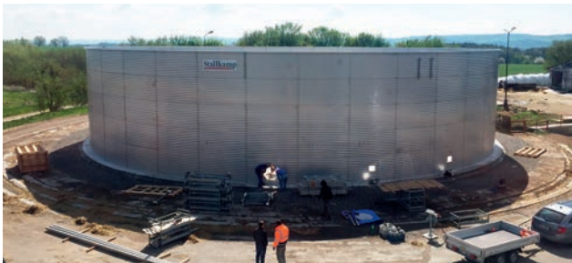
6.283 m 3 Wellstahlbehälter in Tschechien 6,283 m 3 Corrugated steel tank in the Czech Republic
