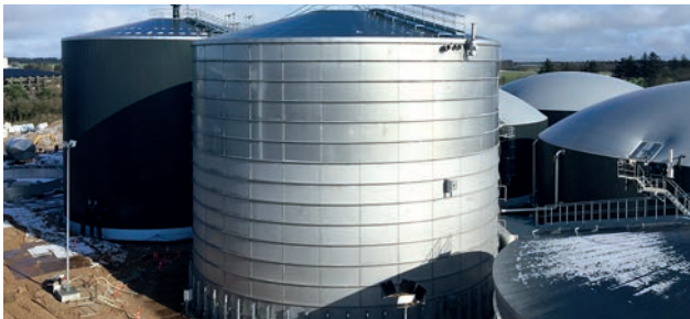
Drei zentralgerührte Fermenter im Bau Three continuous stirred tank reactors during construction
