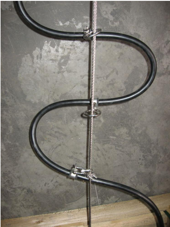
Fig. 7: Cable guide on the wire cable
