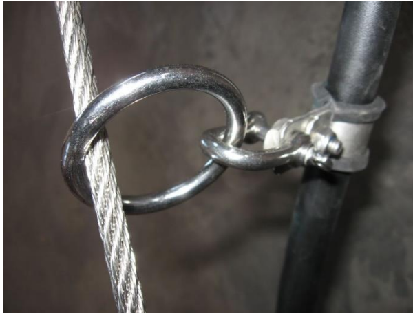
Fig. 3: Cable clamp with shackle and ring
