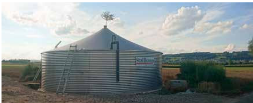
膜屋顶侧视图 | Tank view outside with membrane roof
