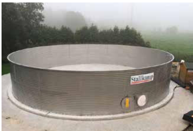
572 m 3 波纹不锈钢板的污水储存罐 572 m 3 Waste water storage made from corrugated steel
