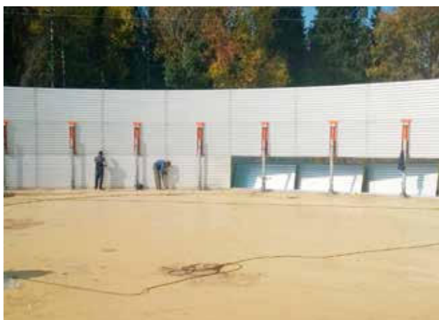
带升降装置的组装现场 Assembly with lifting gear
