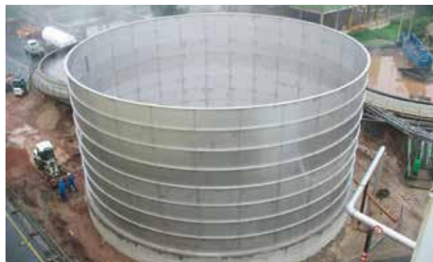
1,661 m 3 造纸厂的污水储存罐 1,661 m 3 Waste water tank for the paper industry
