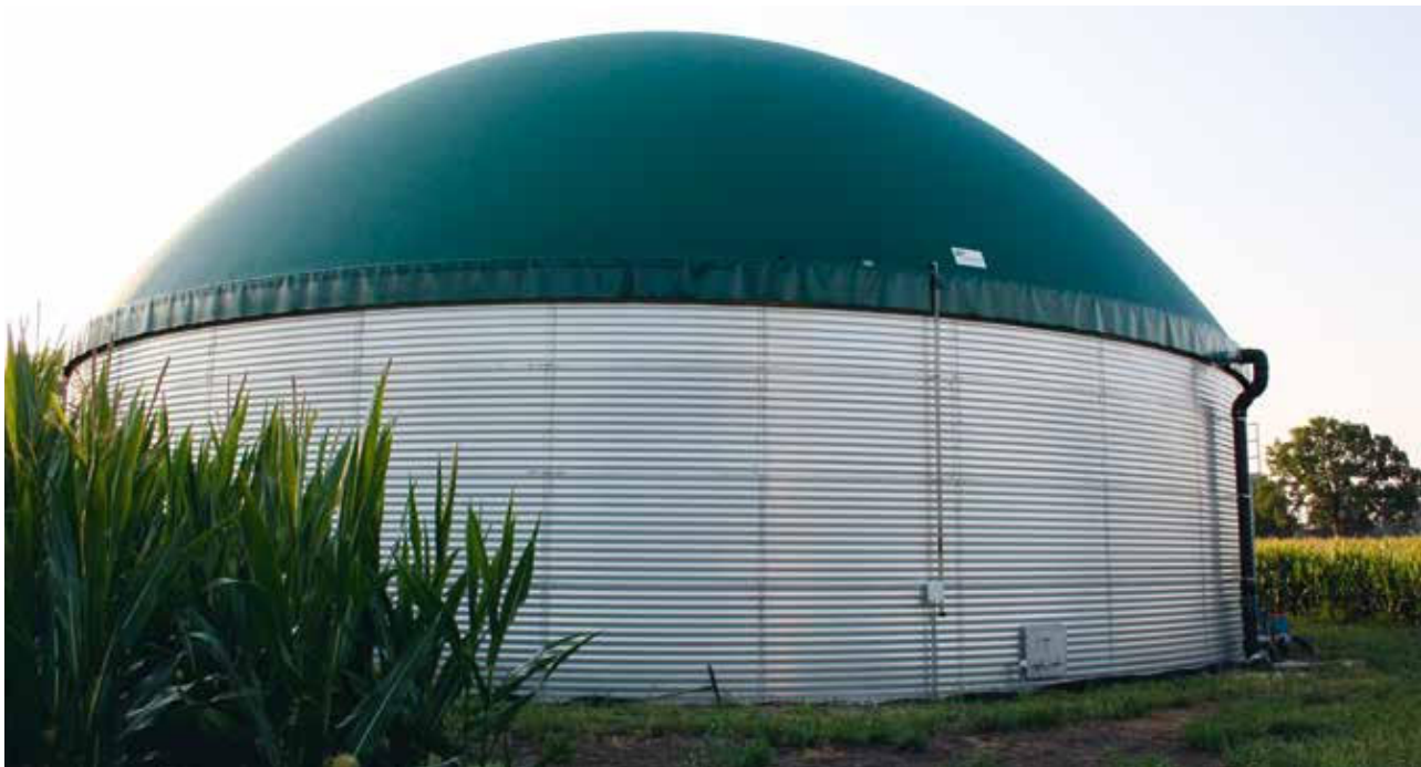
采用气密双层膜屋顶的沼气发酵罐 | V4A biogas tanks with gas-tight double membrane roof
