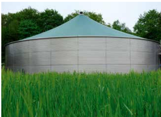
带膜屋顶的波纹不锈钢储液罐 Corrugated steel tanks with a membrane roof
