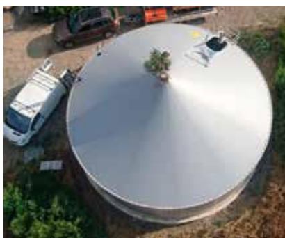
膜屋顶俯视图 | Membrane roof from above
