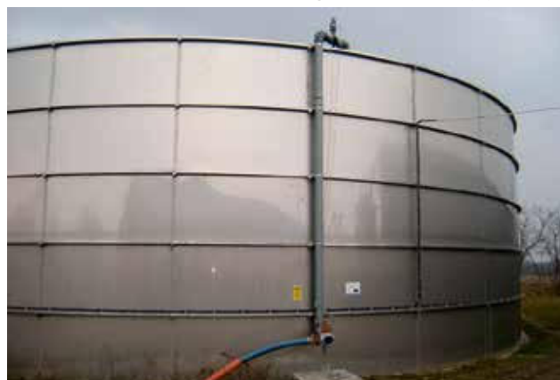
罐侧边的泵送系统（泵入和泵出） Suction and filling station above tank edge
