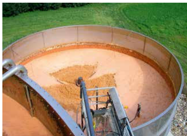
污水罐 Waste water tank
