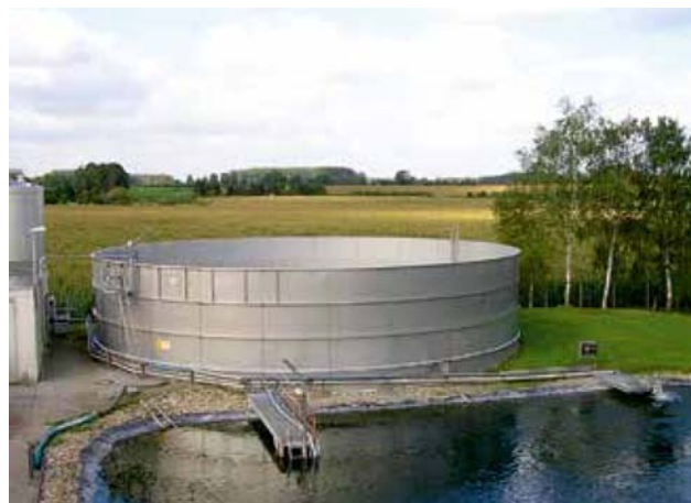
不锈钢污水罐 Stainless steel tank for waste water
