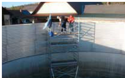
混凝土罐上加高的两圈罐 2. Ring on concrete tank
