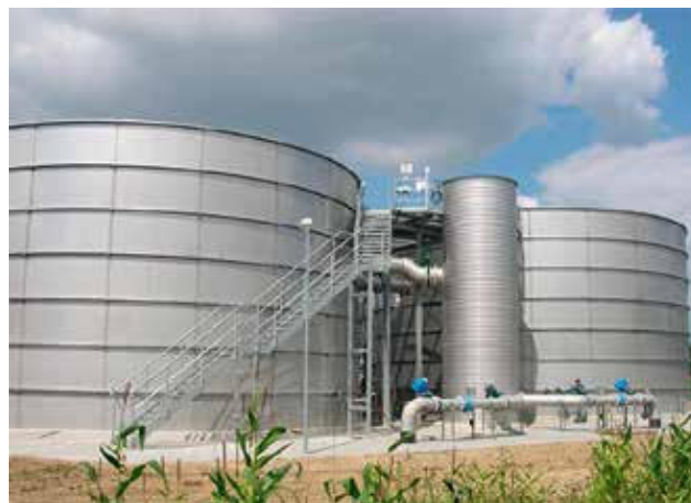
1,664 m 3 平板不锈钢罐和51 m 3 波纹不锈钢罐——造纸厂 1,664 m 3 Stainless steel tank and 51 m 3 corrugated steel tank in the paper industry
