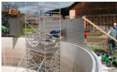
混凝土罐体加高 Adding height to a tank
