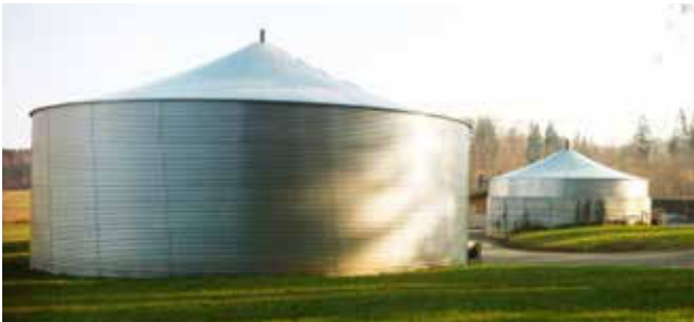
波纹不锈钢罐和混凝土增高罐 (波纹不锈钢) 罐 Corrugated steel tank and heightened concrete tank with corrugated steel tank
