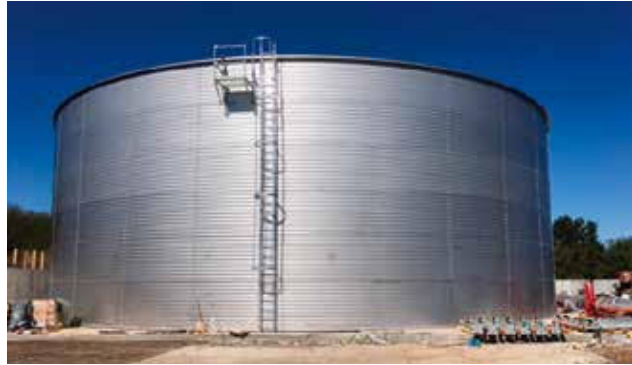
4,230 m 3 粪尿储存罐 (保加利亚) 4,230 m 3 One out of 17 manure tanks in Bulgaria
