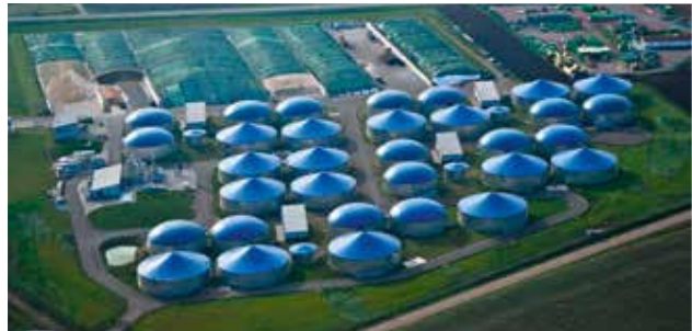
沼气发酵罐, 二级发酵罐和沼液储存罐 Digester, secondary digester and end storage of digestate of a biogas plant
