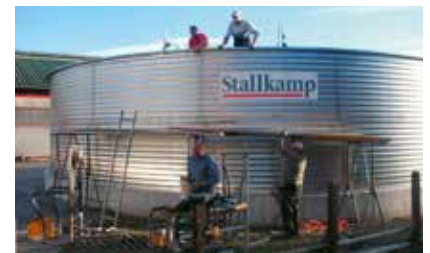
加高后的混凝土罐 Heightened concrete tanks
